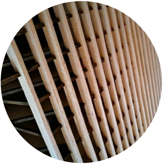
EARLY ROOF STRUCTURE SYSTEM INTEGRATED INTO RAMMED EARTH WALLS
