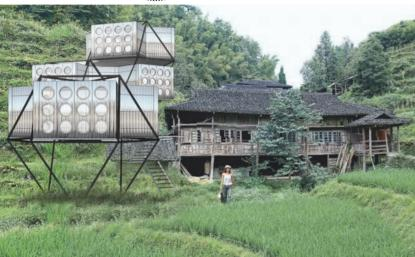
The Plugin Towers were primarily design to circumvent strict planning regulations in Shenzhen, China. This is done through the elimination of foundations. The structures dually are then able to perform in rural areas where casting large foundations may not be possible. The low-cost nature of the structure and ease of assembly makes these structures a system of convenience. (Grozdanic, 2017)
