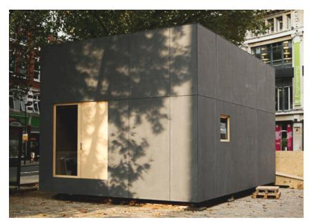
Wikihouse is an open source structure design system, allowing for quick fabrication and assembly of homes. The Wikihouse project is a collaborative effort including; architects, designers, engineers, inventors, manufacturers and builders. Through collaboration the Wikihouse project aims to develop "the best, simplest, most sustainable, high-performance building technologies, which anyone can use and improve." (WikiHouse, 2017)
