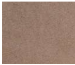
Fig. 8.21. Existing sanblasted concrete
