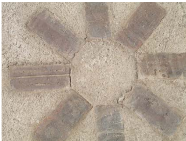
Figure 183: Existing surface detailing found on site.
