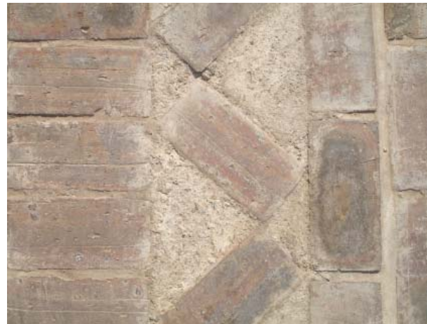
Figure 184: Existing surface detailing found on site. (2)
