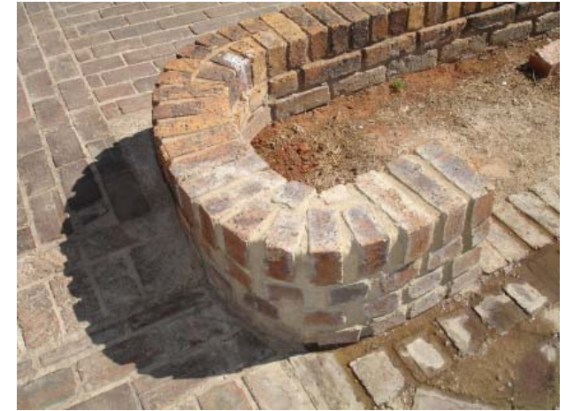
Figure 197: Existing curved brick wall on site.
