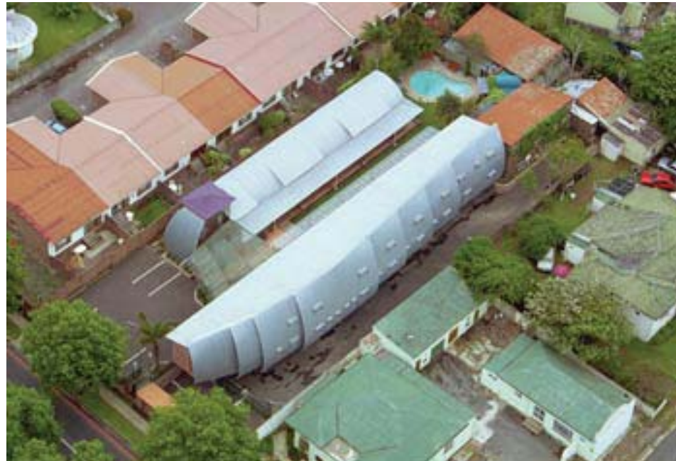
Figure 156: Aerial view of guest house.
