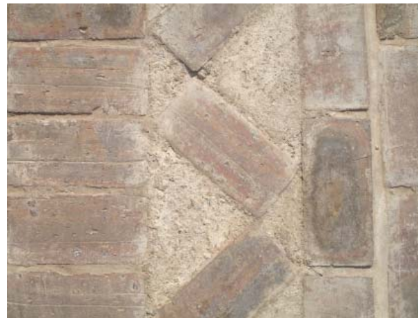
Figure 184: Existing surface detailing found on site. (2)
