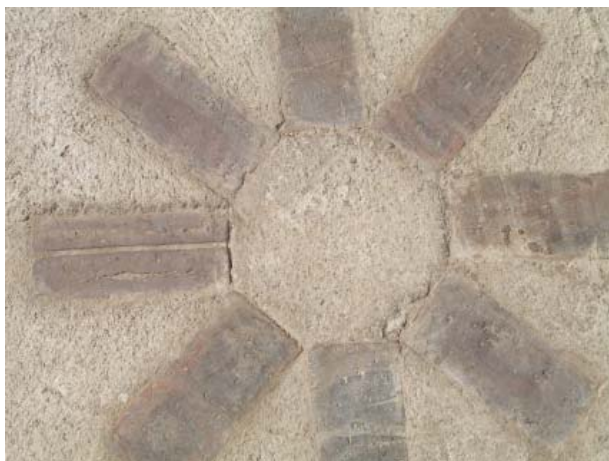
Figure 183: Existing surface detailing found on site.
