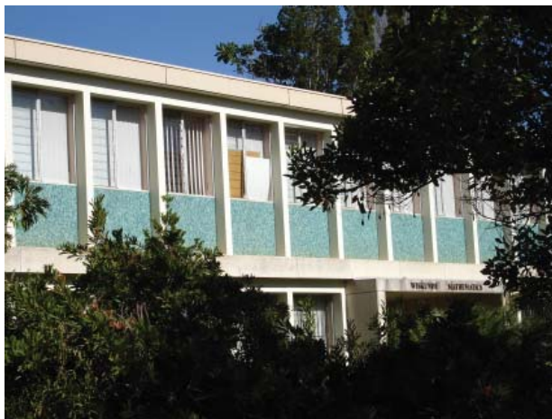
065 The Mathematics buildings (Old Administration) was designed by Gordon Leith and completed in 1931 in the Mannered Neo-Classicism style. Figure 89 (Fischer 1996)
