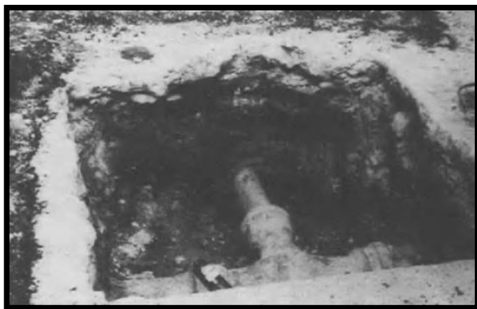
Figure 1: Early Cast-Iron Pipes. (Kramer, McDonald & Thomson, 1992: 20).
