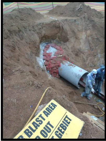
Figure 9: Pipe Jacking of the 900mm pipe (Author's Own Source).
