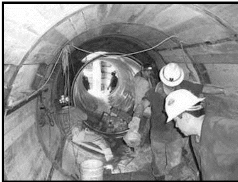
Figure 18: Utility Tunnelling (Water World, 2006: online).
