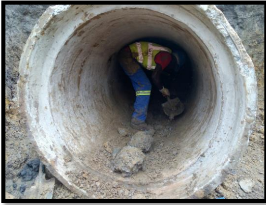
Figure 12: Worker inside 1200mm diameter pipe (Author's Own Source)
