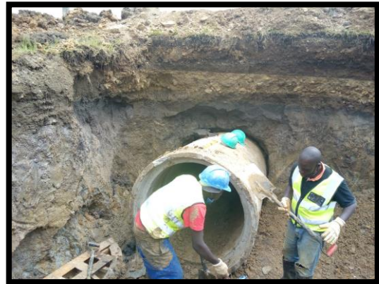
Figure 11: 1200mm diameter pipe being jacked (Author's Own Source).
