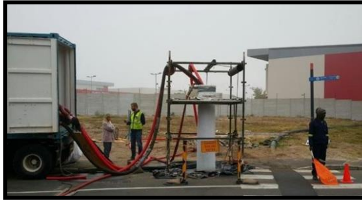
Figure 56: The Sanddrift Project done by AECOM in Cape Town using CIPP (Bizcommunity, 2019: online)
