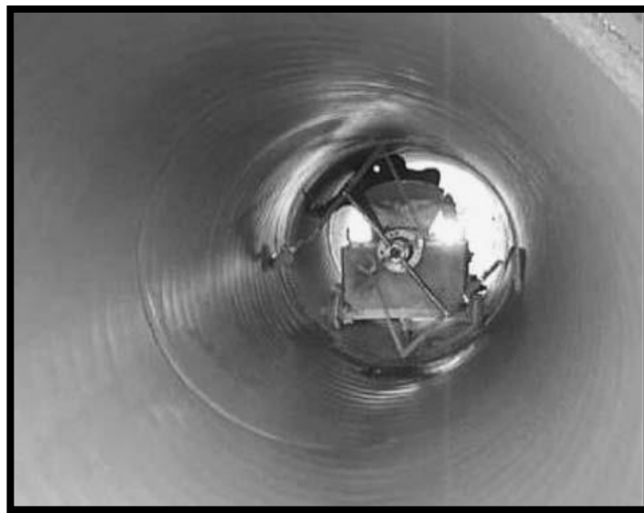
Figure 25: Slip Lining Process (Najafi, 2010: 107)
