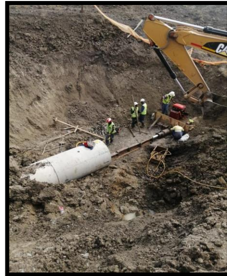
Figure 10 : Final Day of Pipe Jacking for 900mm pipe (Author's Own Source).
