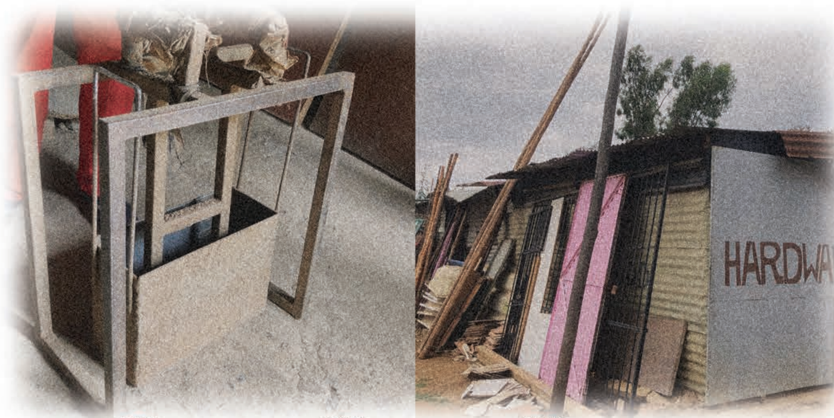
Hardware Stores and Brick Manufacturing Facilities in Melusi (Author 2024)
