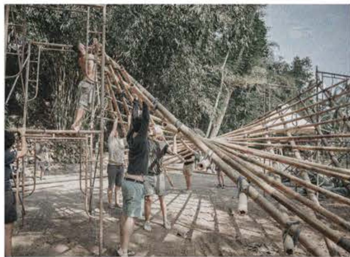
Building Process of Hyperbolic Paraboloid (Bamboo U, 2022)
