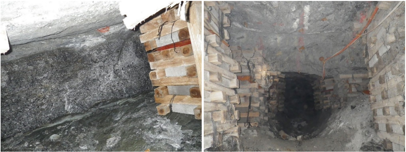
Fig. 2 Typical conditions in the face area of a deep tabular stope with the gold reef shown on the left. The centre gully of the stope is on the right. The dip of the reef can be seen on the left and is approximately 25^\circ
