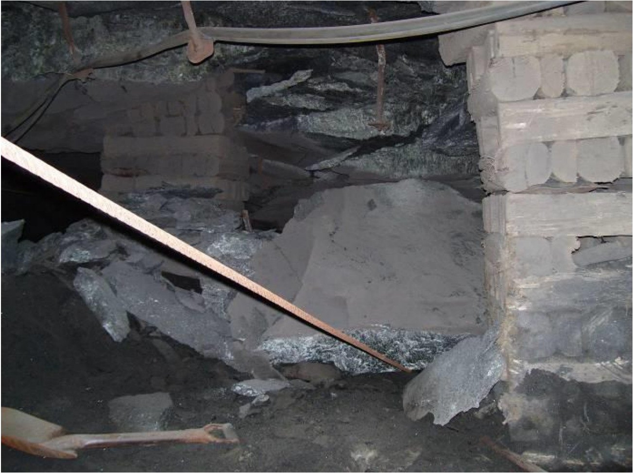
Fig. S7. Collapse in Panel 7N on 04 April 2007.
