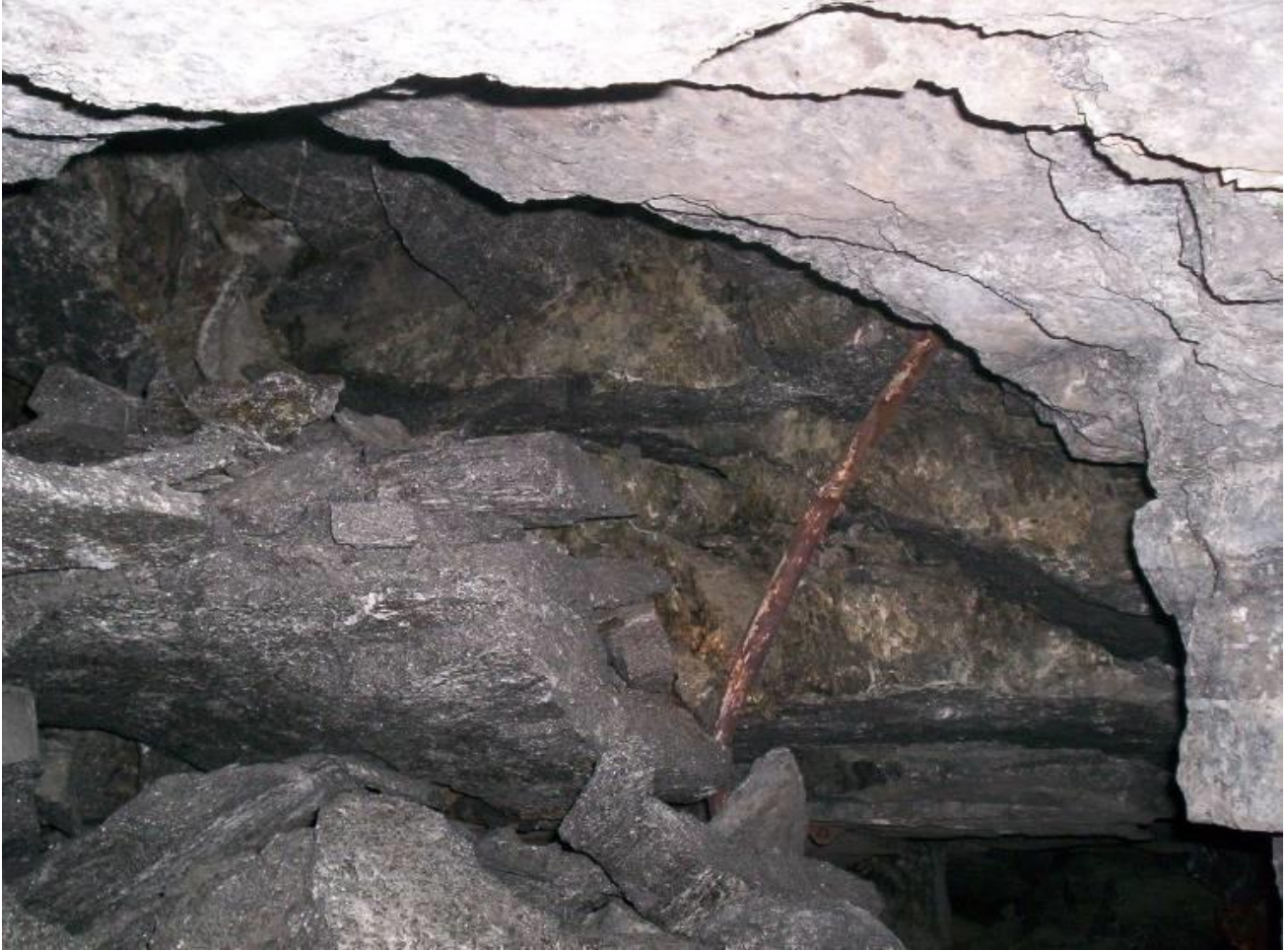
Fig. S6. Collapse in Panel 5S on 17 October 2005.
