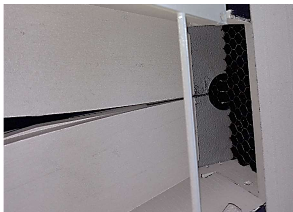
Figure 4.45. Close-up view of coax-to-waveguide launcher and flared waveguide interface.
