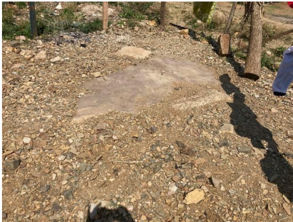
Figure 10: Floors of the shacks that were washed away
