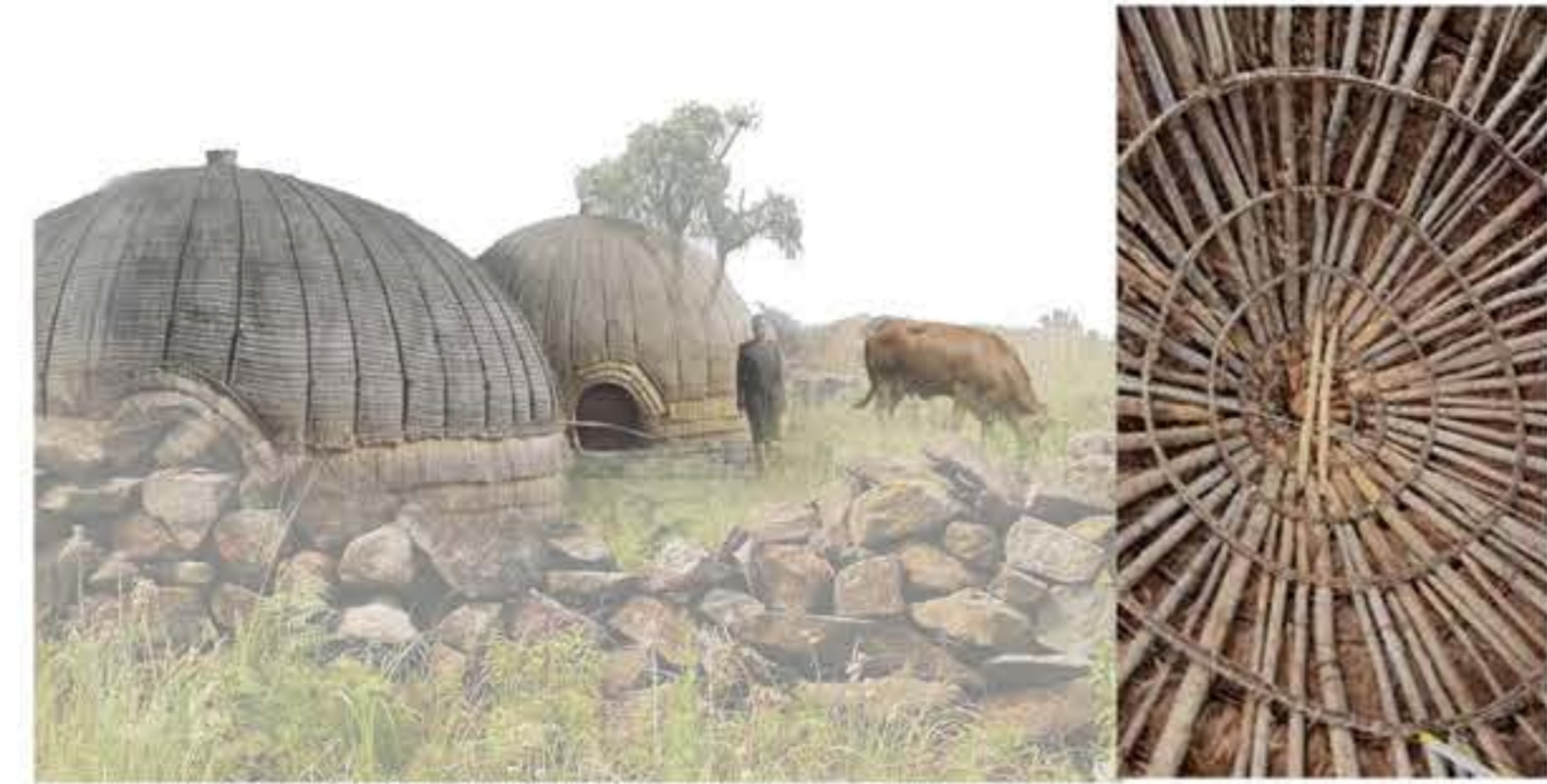
DRY JOINERY TIMBER AND REED DWELLING CONSTRUCTION (ADAPTED FROM DU PLESSIS, 2020: 43).
