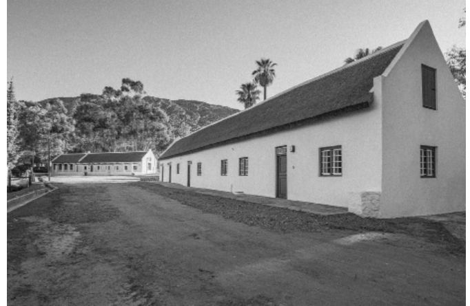
Figure 21: Old school buildings retained and restored as guest accommodation [TV3 Architects adapted by Author 2024].
