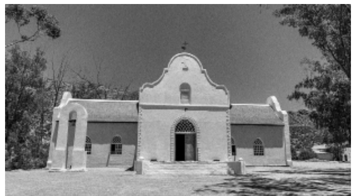
Figure 13: The restored Church in Wupperthal [Tracks4Africa n.d. adapted by Author 2024].
