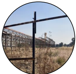
Site (Only 2 x steel structures remaining)
