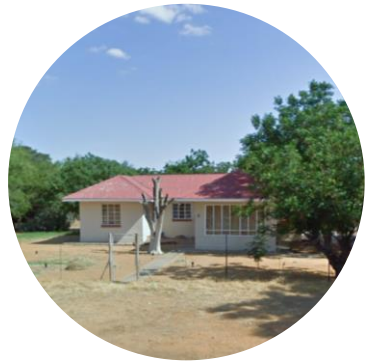
Figure 7: Site and town condition (Author, 2024)
