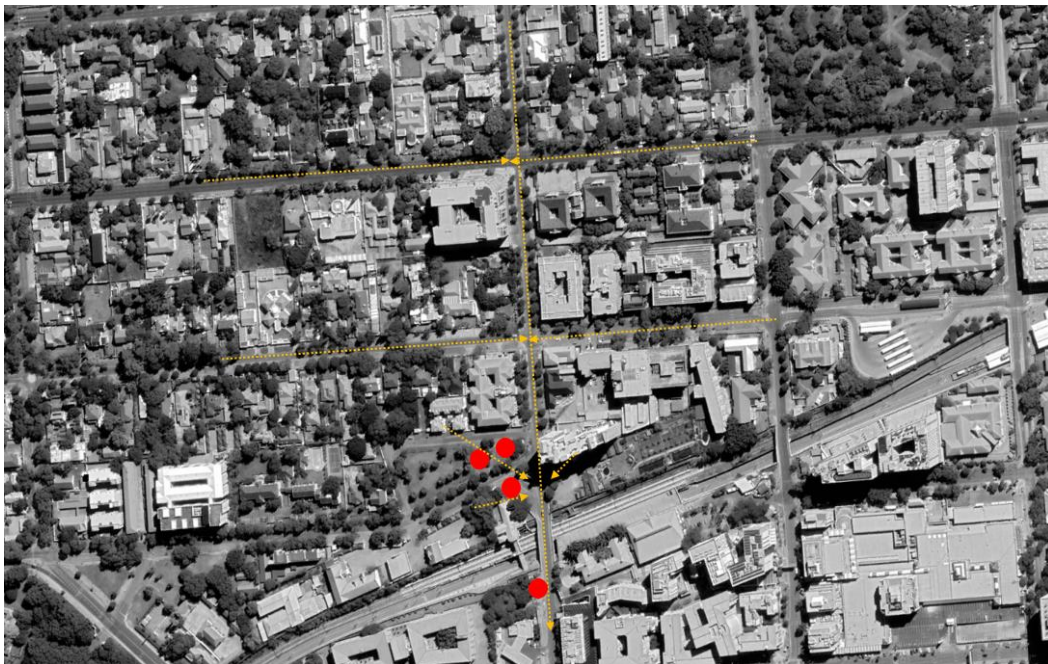
Figure 12: An aerial photograph illustrating Festival Street, pedestrian traffic and strategic location of the informal vendors (Google Earth, 2023).
