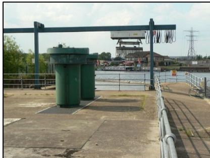
Beeston Hydro on the River Trent (1.66 MW), Nottinghamshire, UK [8]
