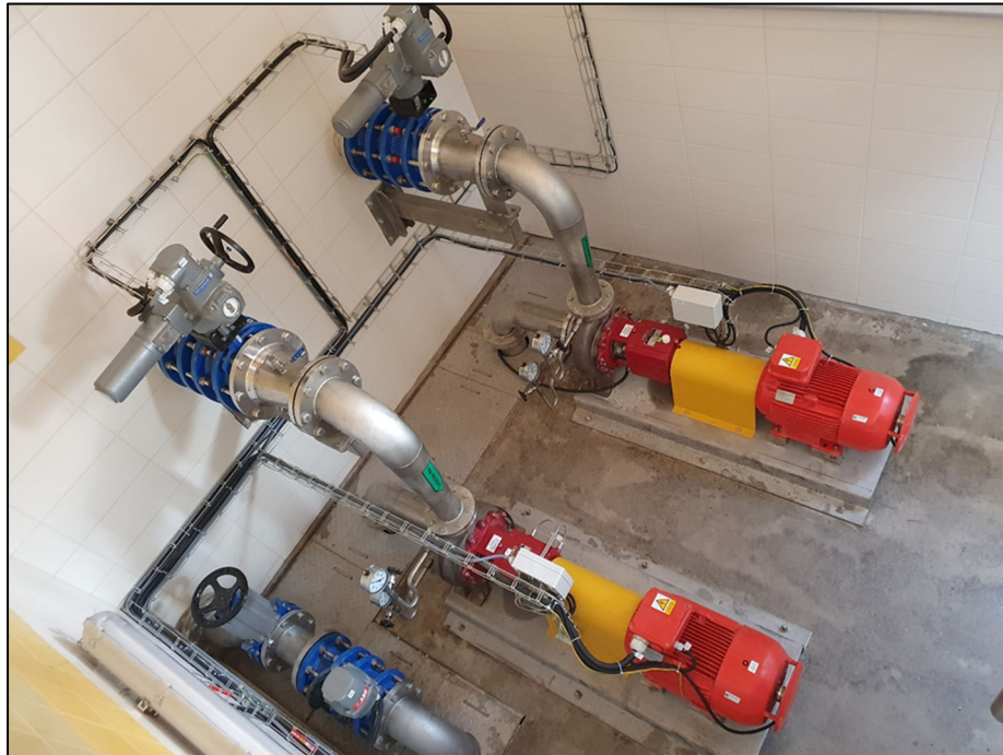
Figure 6: Two pumps in turbine mode (volute one-stage pumps, both rotor and stator parts from stainless steel, mechanical stainless-steel seal, asynchronous generator)
