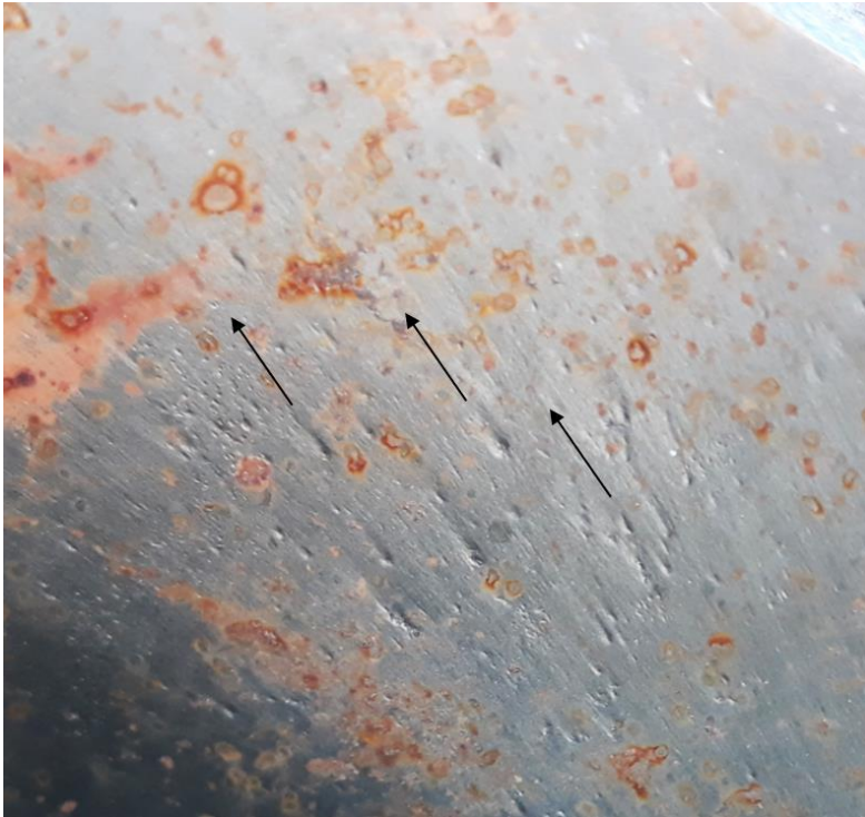
Figure G.1: Wear pattern on spigot of a cast iron dense medium separation cyclone C510-20-0/BB-A/110 (RH) used for diamonds. The cyclone was in use for six months.
