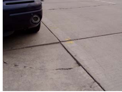
Figure 2b. Corner break destruction in cement concrete pavement
