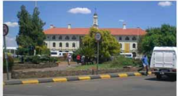
Fig 3.16 The rebuilt Pretoria Station Building in context today, with the Historical Sunken Garden Square in the foreground. (Photo by author)
