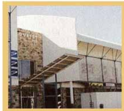
Fig 5.36 A view of the side entrance as seen from the bus rank. (Els 2000)
