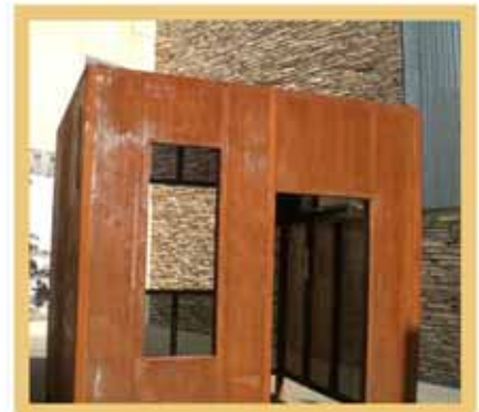
Fig 5.26 A rusting steel audio-visual viewing box set within a small external courtyard adds to the materiality of the building. (photo by author)
