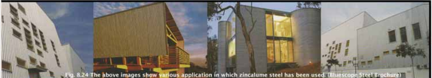
Fig. 8.24 The above images show various application in which zincalume steel has been used. (Bluescope Steel Brochure)
