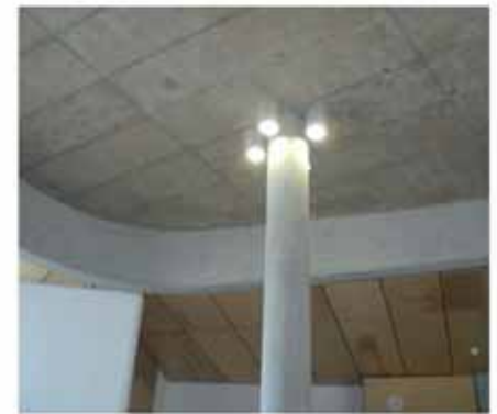
Fig 8.135 The exposed concrete slab of a UP Centenary Building by Earthworld Architects. (photo by author)
