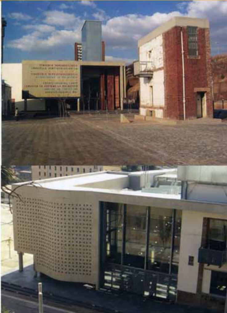
Fig 5.5 above. A glimpse of the roof construction shows how light is diffused through a series of translucent boxes before it enters the foyer area inside. This results in soft, natural lighting effects internally. (Deckler 2006)
