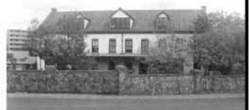
Fig 3.12 The Old NZASM printing store is declared a national monument in 1981 and is therefore protected by Heritage Law. (Photo by author)
