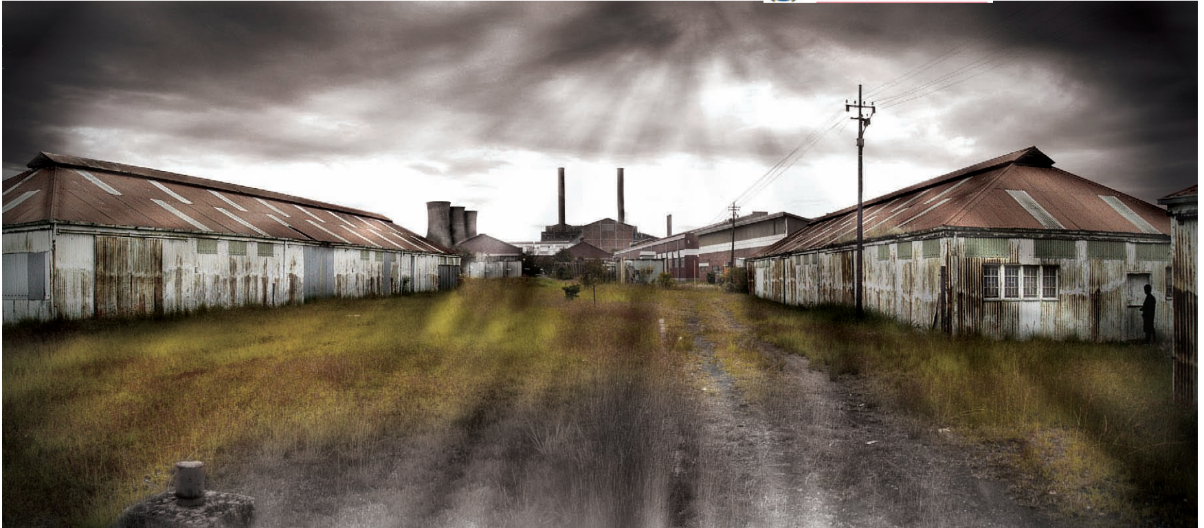
fig. 45 dilapidated warehouses currently on site (view of power station to the West)
