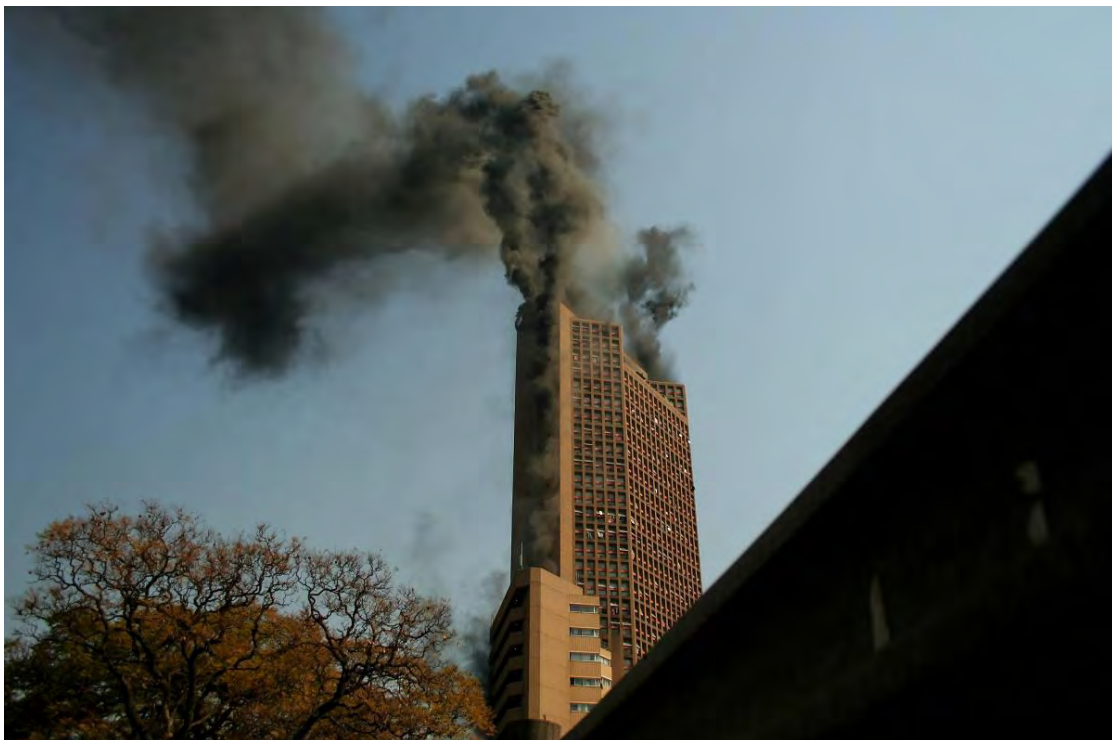
The Kruger Park building on fire (Born, 2008)
