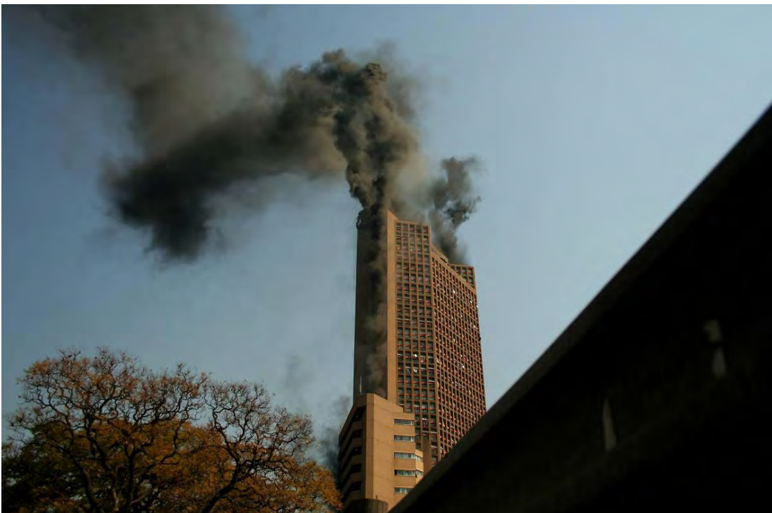
The Kruger Park building on fire (Born, 2008)
