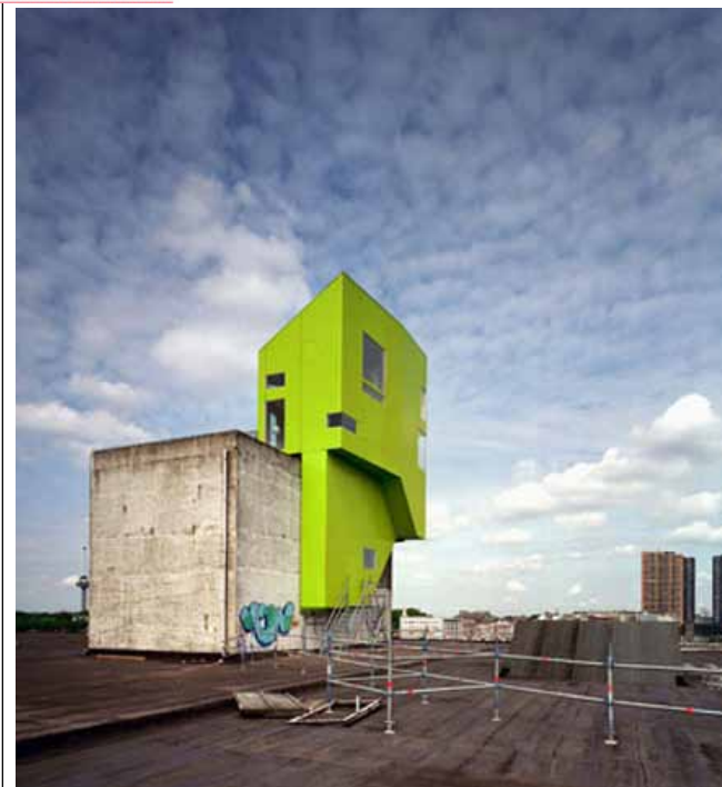
Figure 6.4: View of the Parasite structure
