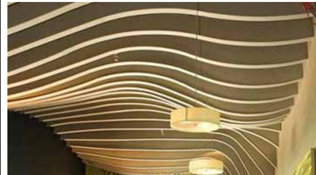
Figure 6.51: Ribbed ceiling view
