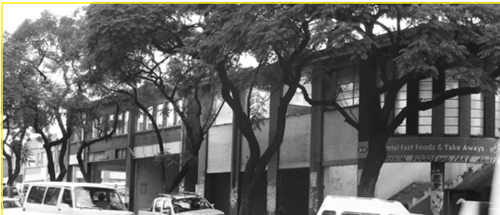
Figure 5.22: View of the east facade
