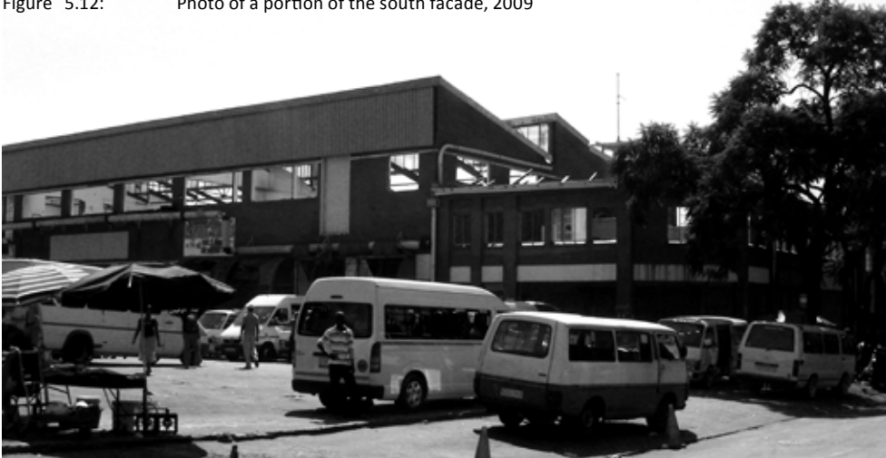
Figure 5.12: Photo of a portion of the south facade, 2009
