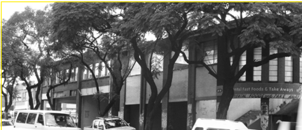
Figure 5.22: View of the east facade
