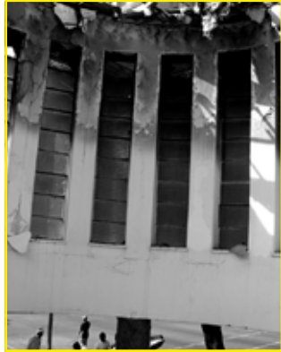
Figure 5.10: Fire damage
